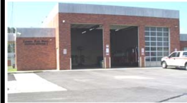
Figure 19: Laurel Fire Stations
