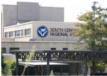
Figure 18: South Central Regional Medical Facility
